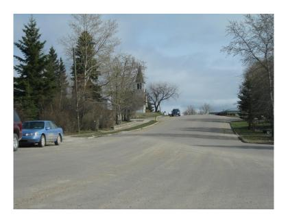
The vertical curve limits driver sight distance in both directions along 10 Street. Limited sight distances increase the risk of head-on, off-road, rear-end and hidden-intersection collisions. Visibility of the 3 Avenue intersection is poor from 1 Avenue at the 1 Avenue/2 Avenue/10 Street intersection because of the intersection alignment, the vertical curve, and the trees along the west side.
