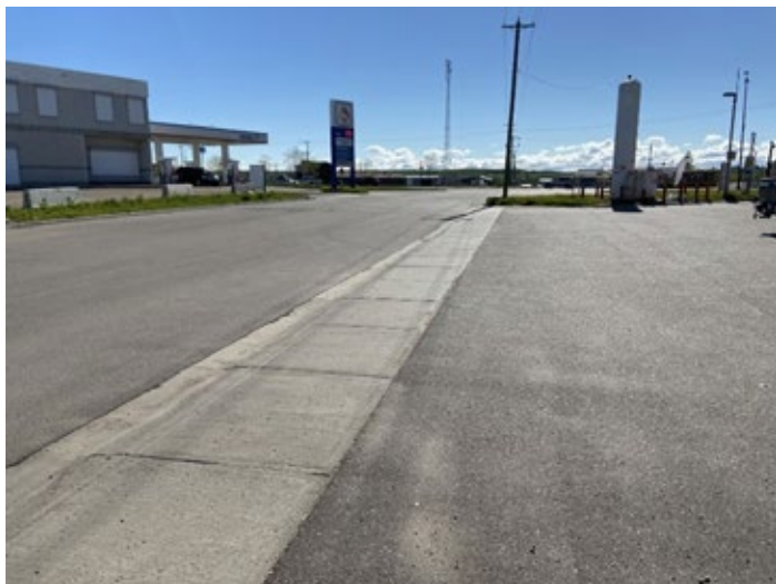
Figure 60: Abrupt trail transition to sidewalk before terminating at 55 Ave (Cold Lake)
