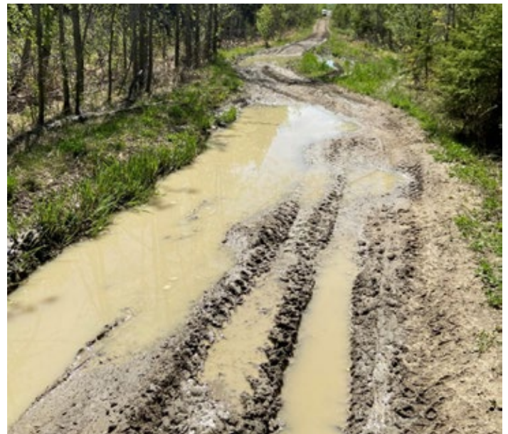
Figure 9: Typical cupped and failing seismic line following recreational use
