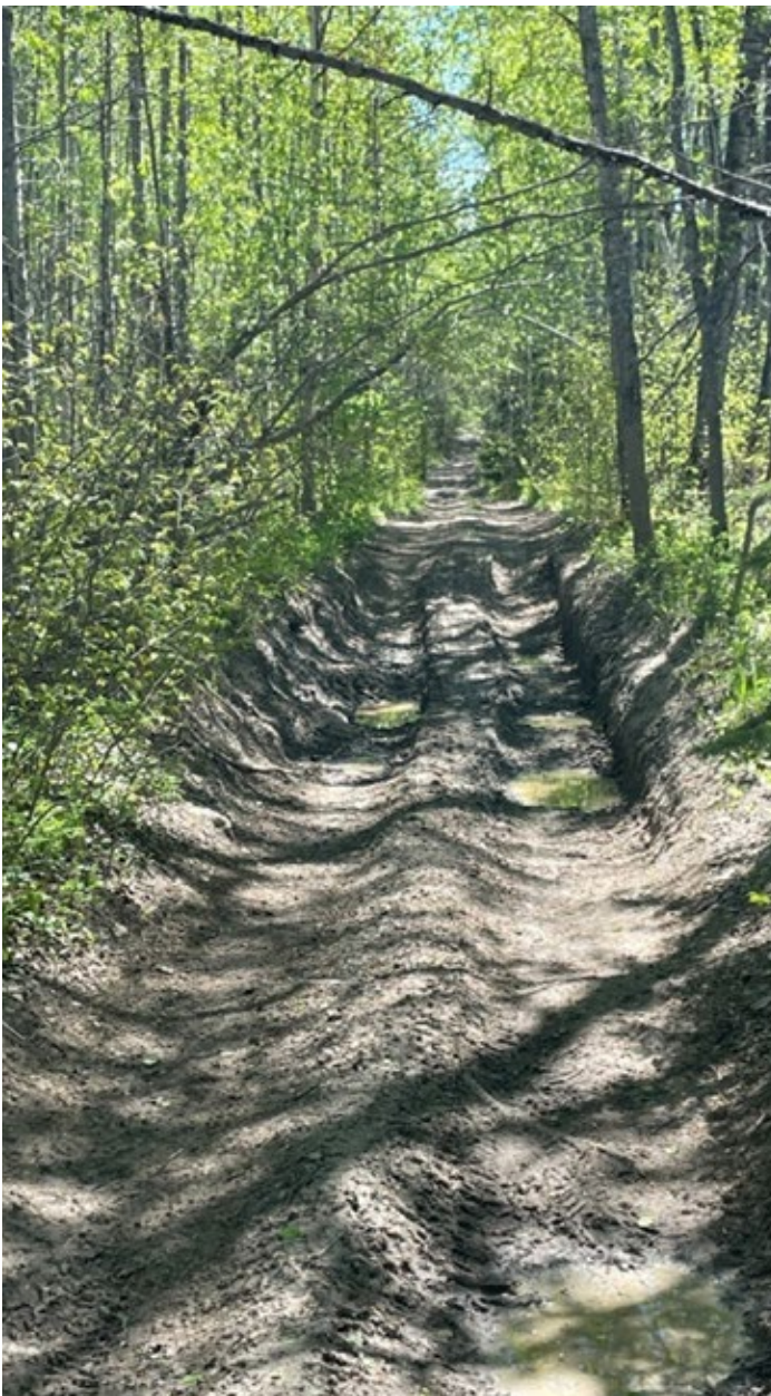
Figure 8: Typical cupped and failing seismic line following recreational use
